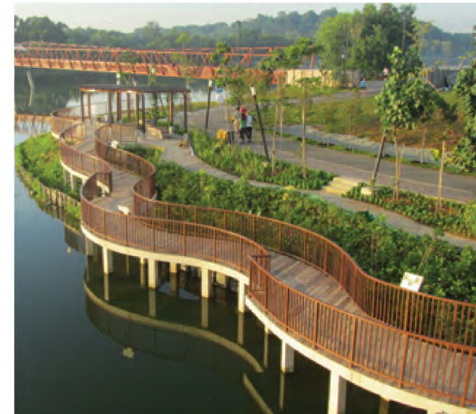
PUNGGOL WATERWAY, SINGAPORE
